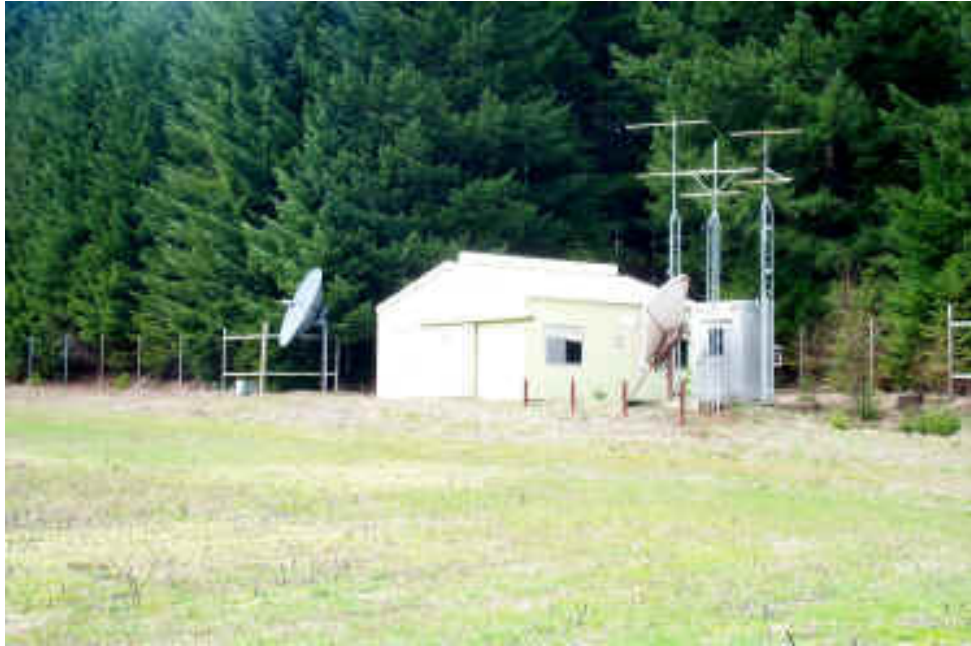
VIEW OF CHEMICAL STORAGE BUILDING 2324 LOOKING NORTH
